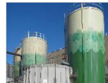
Torres (Spain, winery) 650 m 3 /d
