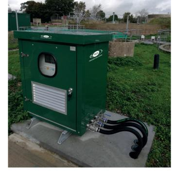
te-sewpas<sup>TM</sup> is available as a 1, 2, 3 or 4 way unit, with individual on/off control. Manual operation is also available for instant desludging when required.
