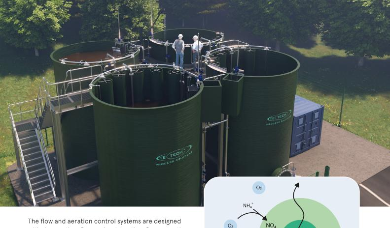
The flow and aeration control systems are designed with dry weather flow and wet weather flow operating protocols as standard, with maintenance cycles available with 3 or more parallel reactor basins. The transition between cycles, whether automatic or manual, is done via the PLC system without affecting the continuity of the plant operation.
