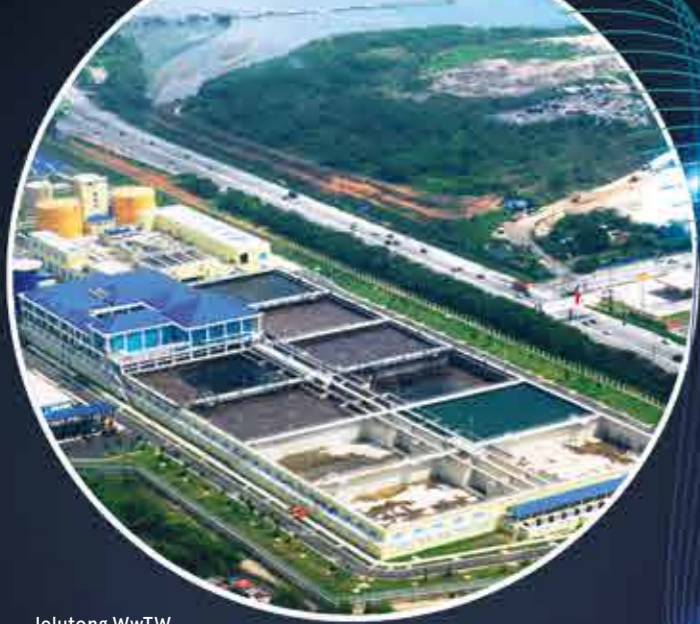
Jelutong WwTW Malaysia, 1.2million PE
